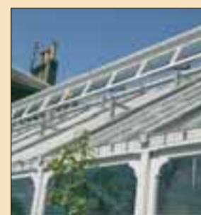
Greenhouse refurbishment at Turriff Nurseries.
